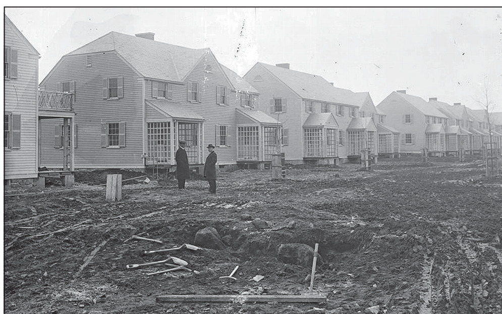
Project 157 homes, left, are shown under construction in this photo from 1918 or 1919. JOHN RUDDY
